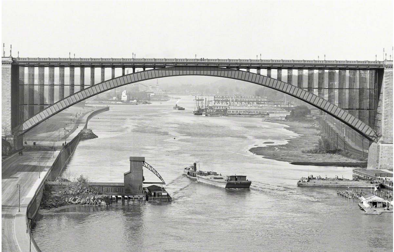
Figure 1. Northward view of Washington Bridge spanning Harlem River, c. 1905. The Morris Heights yard of Charles L. Seabury Co. and Gas Engine & Power Co., Consolidated is visible in the distance on the east side of the river. (Source: Shorpy.com, http://www.shorpy.com/node/19992 .)
